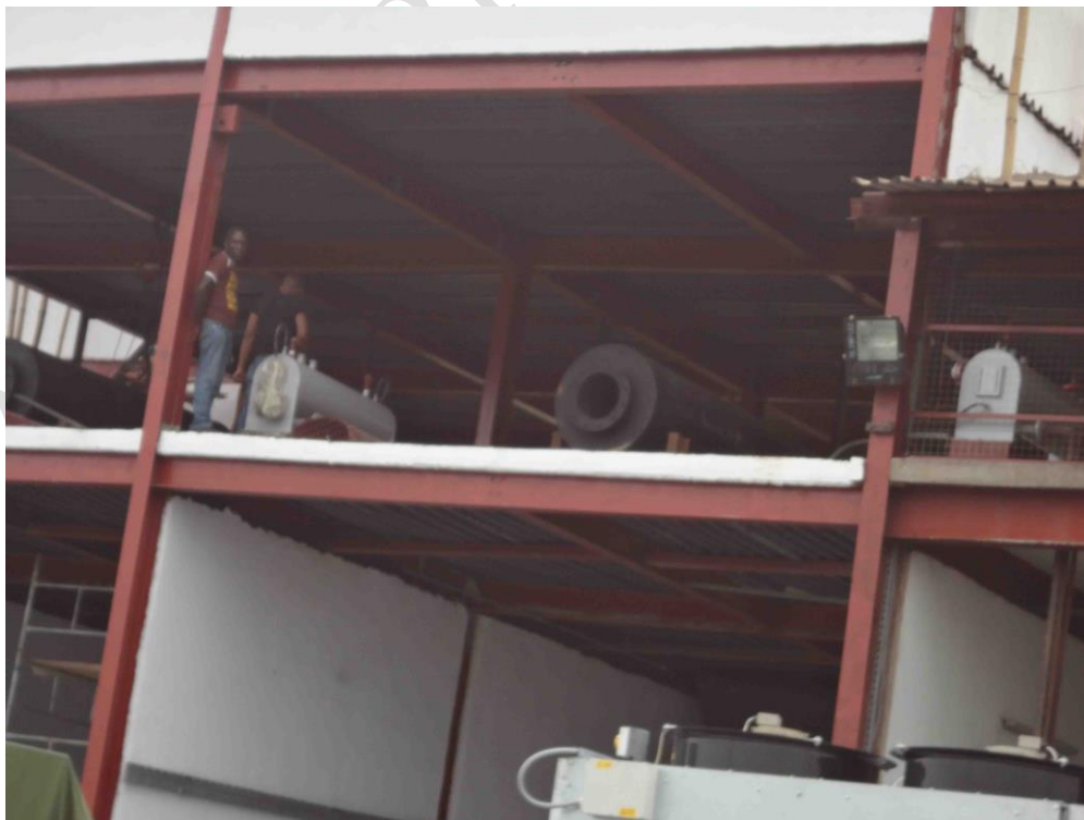
COMPOSITE FLOOR SYSTEM OF CONSTRUCTION FOR MEZZANINE FLOOR OF ISOLO POWER GEN. LTD. ISOLO, LAGOS STATE.
