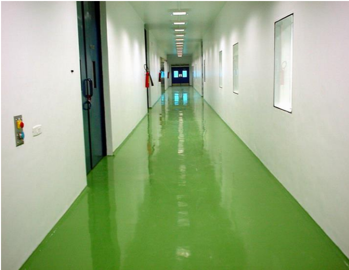
EPOXY FLOOR FINISHING ALONG AISLE FOR RANBAXY NIG. LTD.
