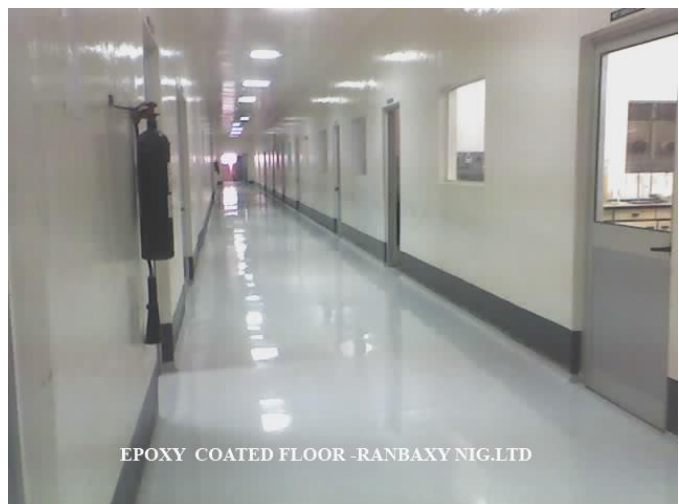
EPOXY FLOOR FINISHING ALONG AISLE, AT RANBAXY NIG. LTD.
