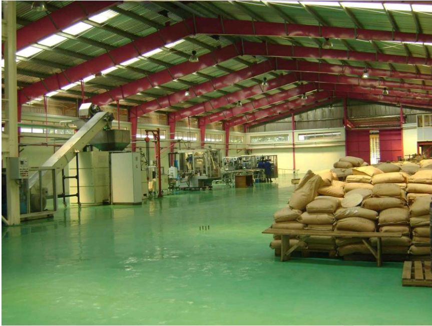
EPOXY FLOOR FINISHES OF FACTORY BUILDING FOR RECKITT BENCKISER, AGRARA, LAGOS STATE.
